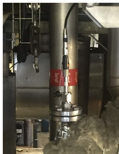
Fig. 6: Installation of the probes into transfer lines of the boiler and condenser of a batch distillation plant.
