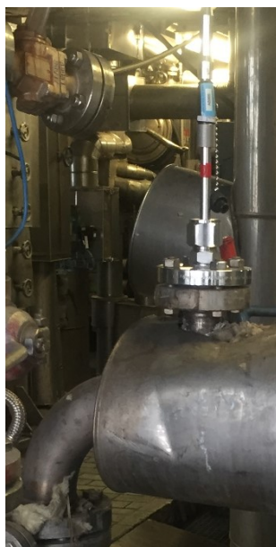
Fig. 6: Installation of the probes into transfer lines of the boiler and condenser of a batch distillation plant.
