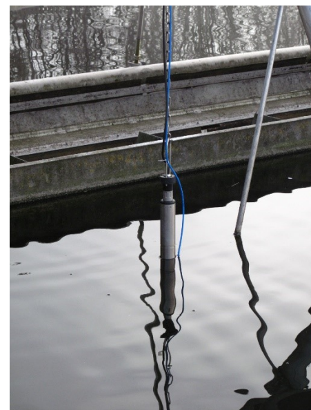
Fig. 3: Installation of the NiCaVis® 705 IQ sensor in the clarifier of the wastewater treatment plant Peißenberg
