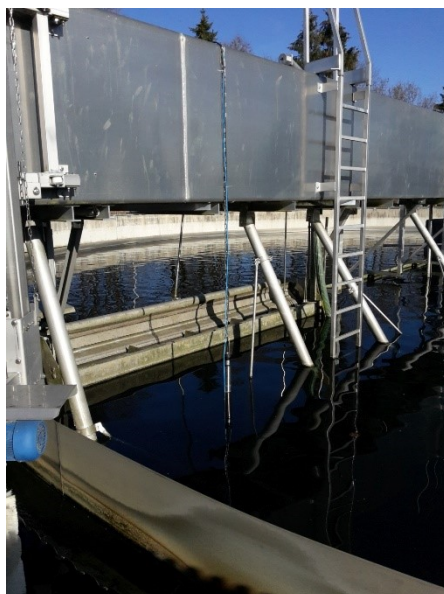
Fig. 3: Installation of the NiCaVis® 705 IQ sensor in the clarifier of the wastewater treatment plant Peißenberg
